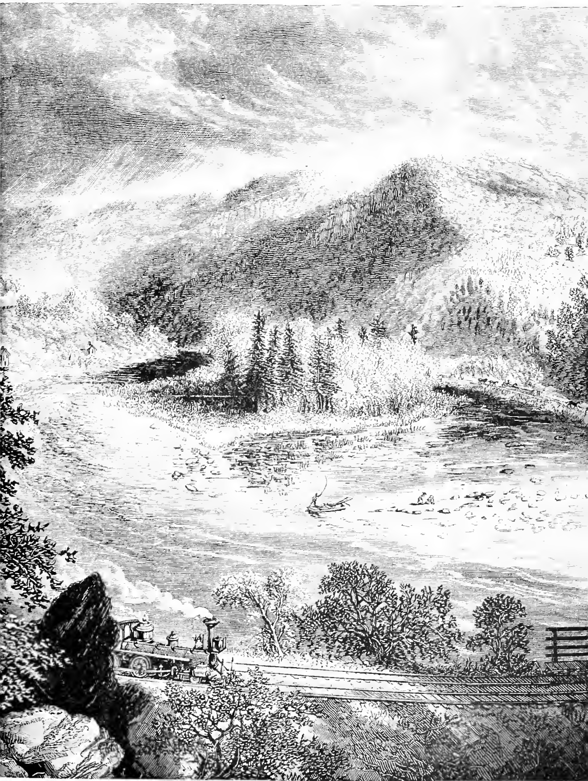
ROCK RIFT ON THE DELAWARE DIVISION ERIE RAILWAY, NEAR PORT JERVIS, N. Y.
